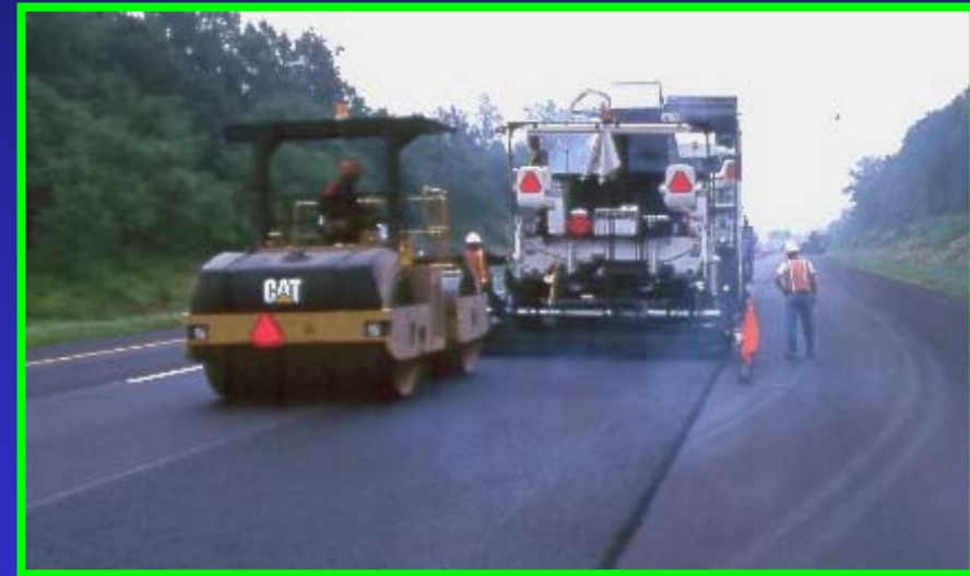
Roll from cold side w/ 150 mm overlap
