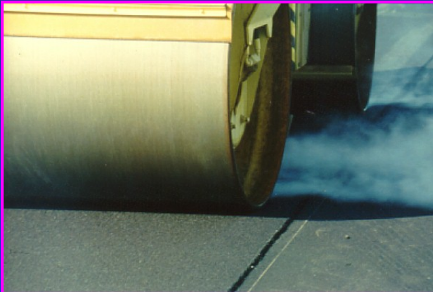
Roll from cold side w/ 150 mm overlap
