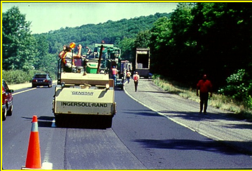
Roll from cold side w/ 150 mm overlap
